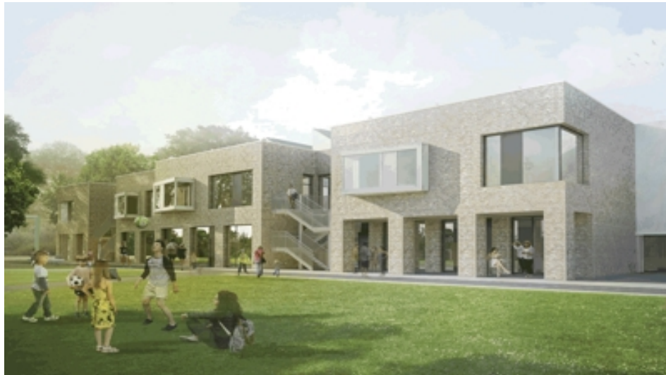
Figure 5: New section of Katrinedals Skole built with reused bricks and cement-free lime mortar
